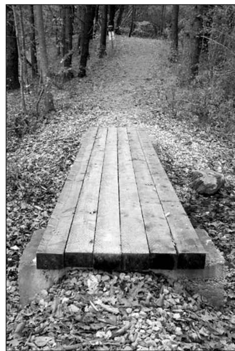
Inset above left is a photo showing remnants of one of the two rotting footbridges on our nature trails that were replaced in spring 2013 by the crew of Steve Pike, Skip Weeks, and Tom Ayres. At left is the new bridge in place, with the robust 4x6s tied together from below and secured to the existing concrete piers. This bridge is located not far into the woods at the northeast corner of the meadow behind the Weeks Brick House. At right is the other new bridge the crew wrangled into place at the beginning of the trail that leads from the parking lot on Tide Mill Road. (If this kind of work is just your kind of non-profit volunteer board service, by all means contact us by phone, e-mail, or postal mail!)
