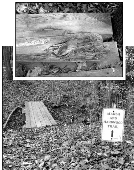
Inset above left is a photo showing remnants of one of the two rotting footbridges on our nature trails that were replaced in spring 2013 by the crew of Steve Pike, Skip Weeks, and Tom Ayres. At left is the new bridge in place, with the robust 4x6s tied together from below and secured to the existing concrete piers. This bridge is located not far into the woods at the northeast corner of the meadow behind the Weeks Brick House. At right is the other new bridge the crew wrangled into place at the beginning of the trail that leads from the parking lot on Tide Mill Road. (If this kind of work is just your kind of non-profit volunteer board service, by all means contact us by phone, e-mail, or postal mail!)
